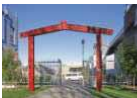
Whanganui UCOL Side entrance pare
